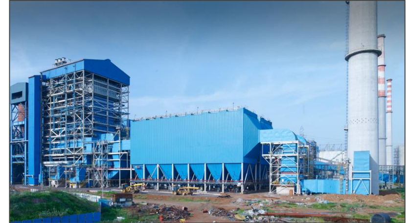
ESP, 180MW Coal based Power Plant for OPG Power, India
