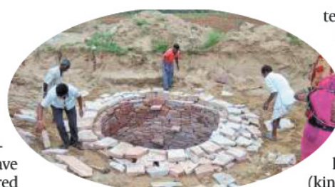
Back to tradition The team hand-dug a deep traditional well, plastered with lime, to store sweet water
