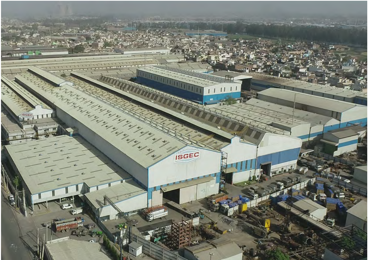
Isgec Plant at Yamunanagar (Haryana) India.
