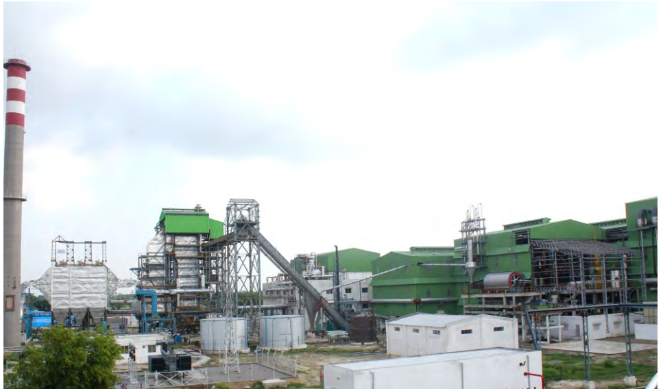
3500 / 5000 TCD Sugar Plant with 15 MW Co-Generation executed on EPC basis including civil works at The Kisan Sahkari Chini Mills Ltd., Sathiaon, Azamgarh, (Uttar Pradesh) India
