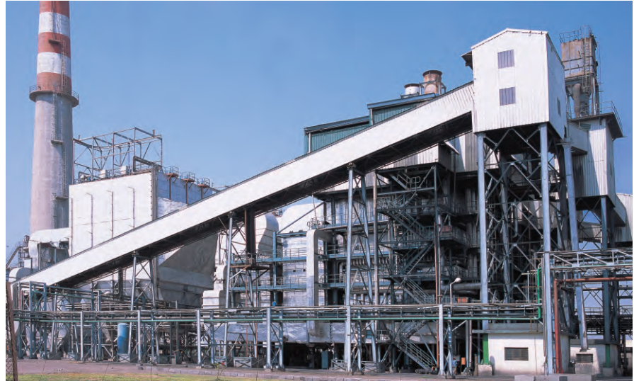
2 x 105 TPH, 67 Kg/sq.cm., 485 Deg.C Coal Fired AFBC Boilers at Rajasthan Spinning and Weaving Mills Ltd., India
