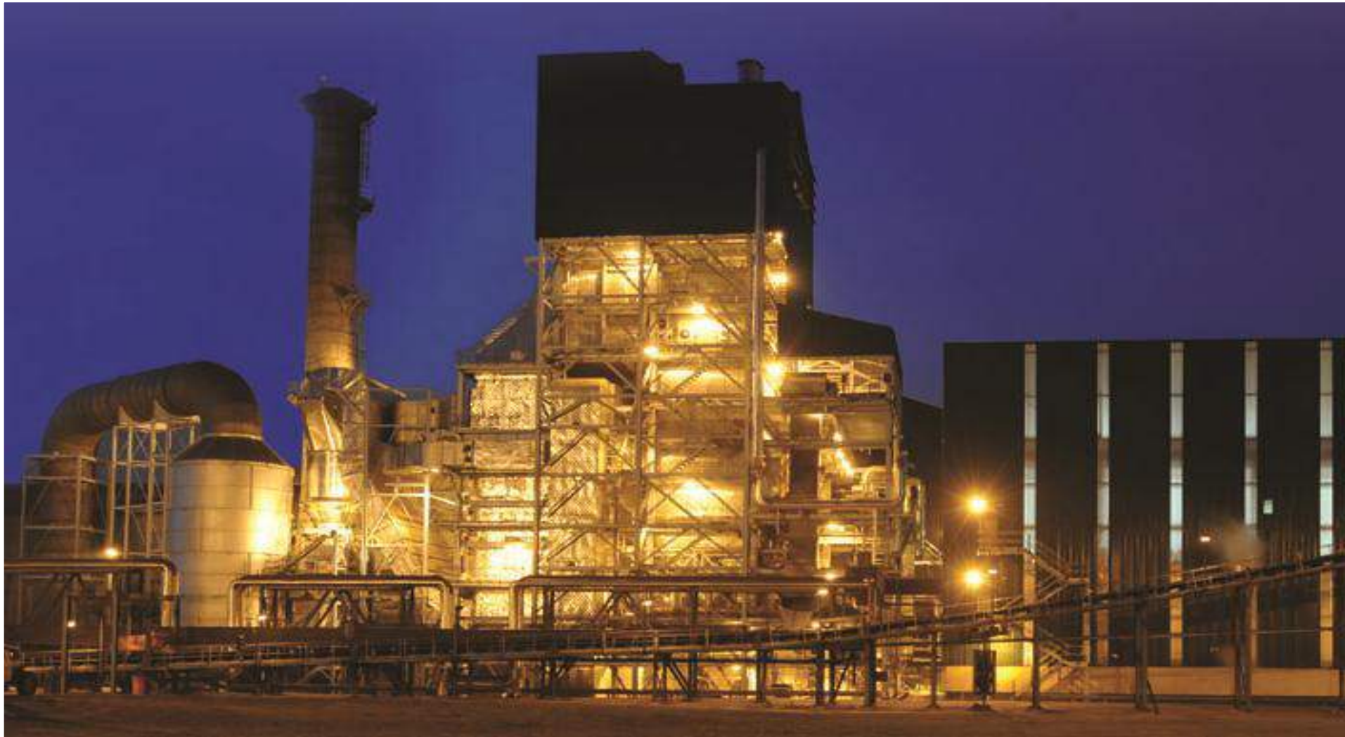
30.4 MW Cogeneration Power Plant
