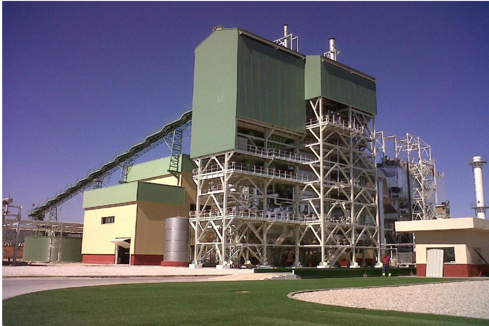
28 TPH Biomass Fired Boiler for 8 MW Power Plant
