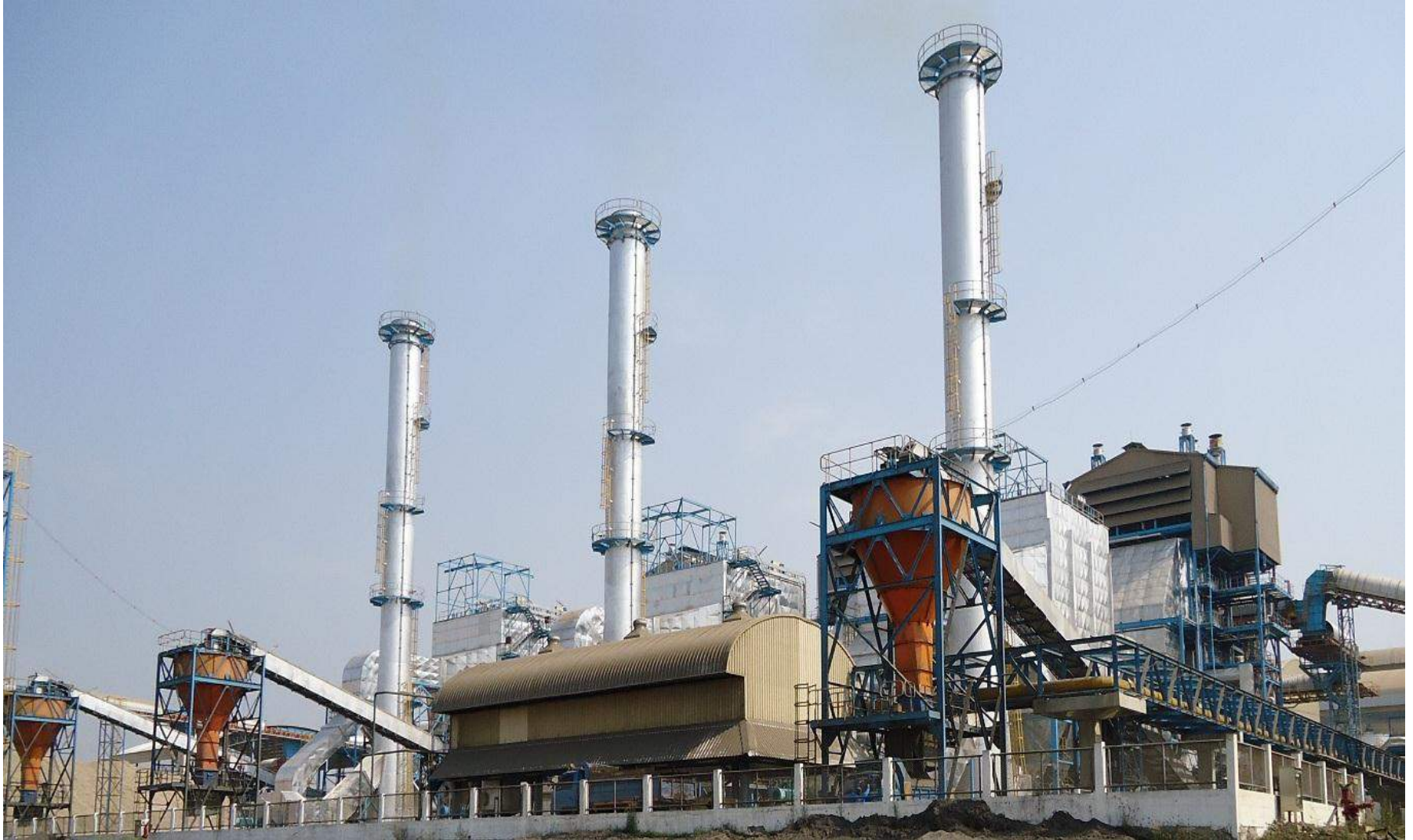
3 x 150 TPH, 40 kg/cm 2 (g), 450 Deg.C Travelling Grate Boilers
