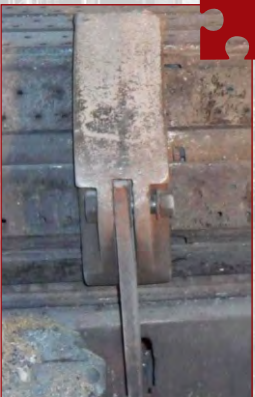
KVK Bioenergy: Travelling Grate Stoker replacement on Walchandnagar Boiler
