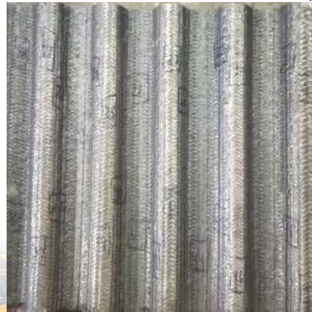
Water Wall Panels Overlay
