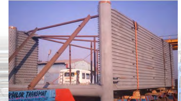
CFBC, Semi Assembled Cross Over Duct
