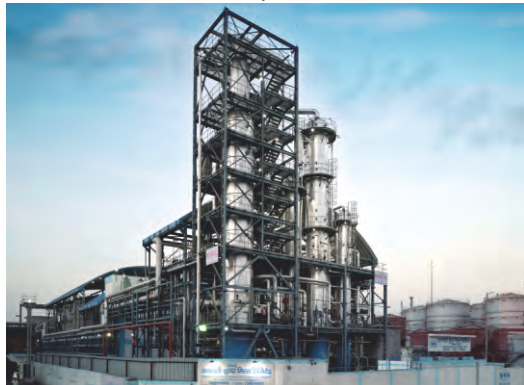
Distillation Section at a Distillery Plant
