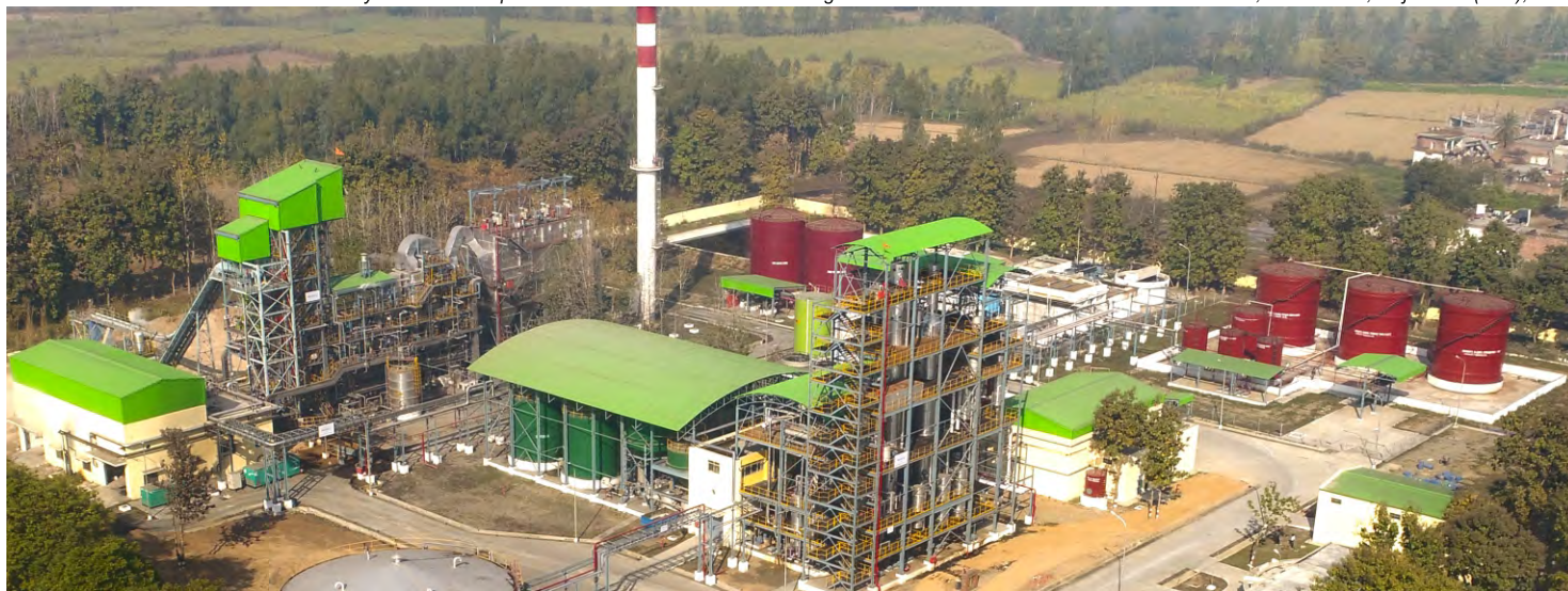
40 KLPD Distillery Plant with Slop Fired Boiler & Power Plant including Civil Work at The Kisan Sahkari Chini Mills Ltd., Sneh Road, Najibabad (U.P.), India
