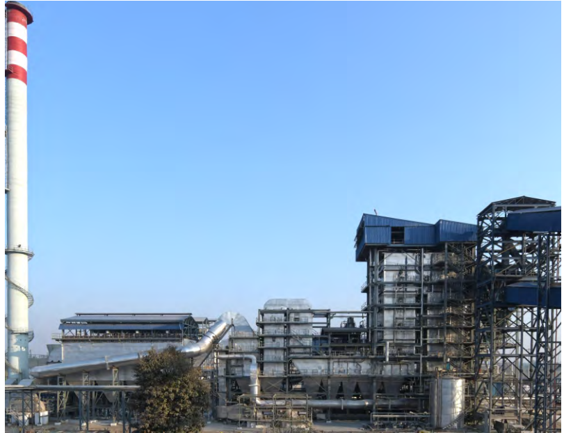
80 TPH, 45 kg/sq.cm. (g), 400 Deg. C, Slop / Bagasse Fired Travelling Grate Boiler at DCM Shriram Sugars, Ajbapur (U.P.), India
