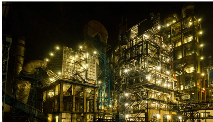
One of the world's largest Cement Waste Heat Recovery Boiler generating 34.5 MW power from a single cement line.
