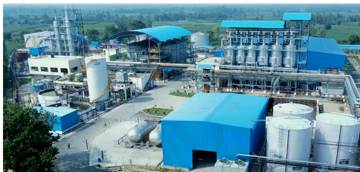
175 KLPD multi-feed Ethanol Plant with 44 TPH Slop Fired Incineration Boiler and 5 MW Power Plant in North India running on fermentation efficiency 93%+ and 115% capacity utilisation.
