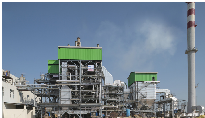
Paddy straw fired high pressure and high temperature water cooled Vibrating Grate Boiler, which reduces 75,000 tons of CO 2 emission by preventing stubble burning.
