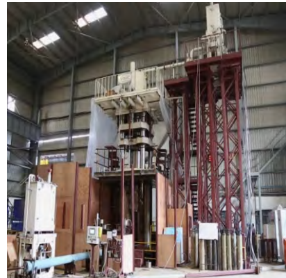
Nuclear Waste Compaction Press
