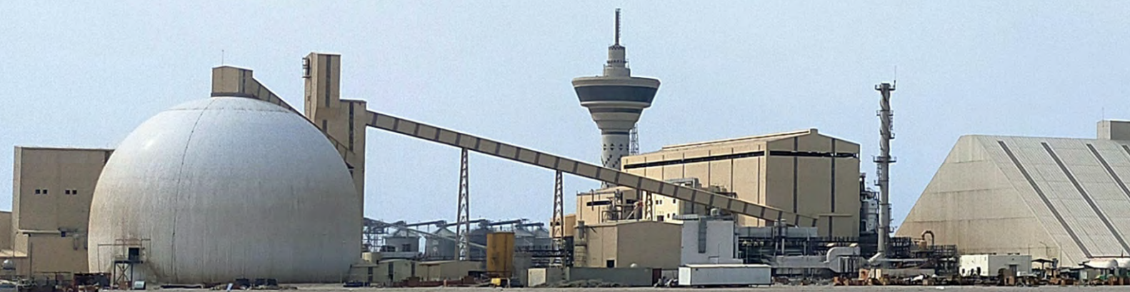
2500 TPD Standalone Port-based Sugar Refinery including 100 TPH Boiler and 12 MW Power Plant at Durrah Advanced Development Company, Yanbu Port, Saudi Arabia
