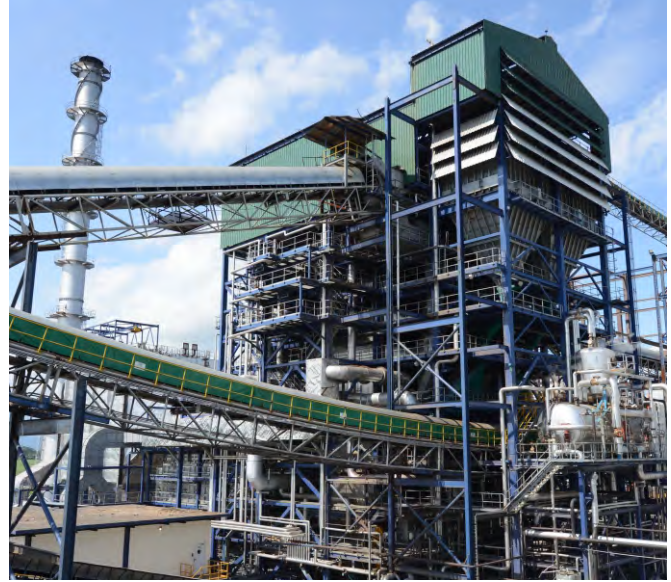
220 TPH, 109 Kg/sq.cm. (g), 540 ± 5 Deg C Bagasse Fired Travelling Grate Boiler at Ingenio Magdalena, Guatemala
