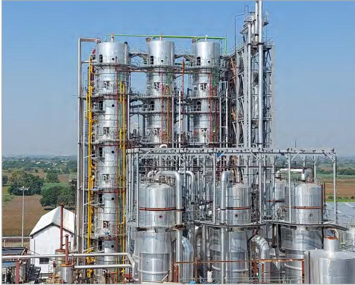
5000 TCD Sugar Plant-A/B/C Boiling Vertical Continuous Pan(VCP) at Twentyone Sugars Ltd., (Unit-1) Maharashtra, India
