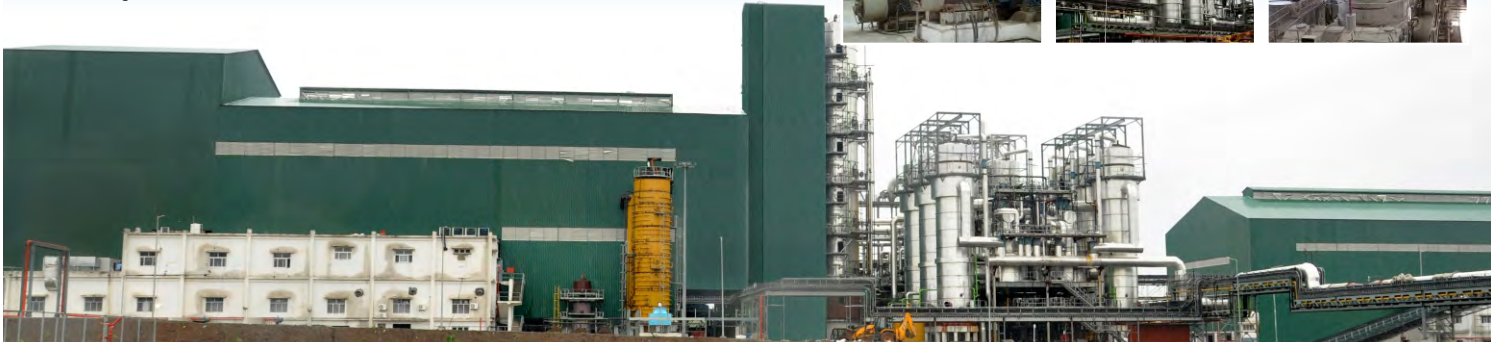
10000 TCD Refined Sugar Plant with 210 TPH / 125 Bar, Bagasse Fired Boiler and 40.5 MW Power Plant, having all FFE & VCP designed on 30% Steam with Refinery at KPR Sugars, Karnataka, India
