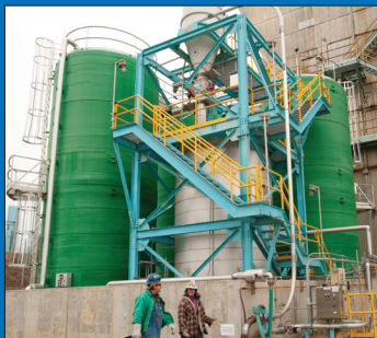
Urea solution storage tank
