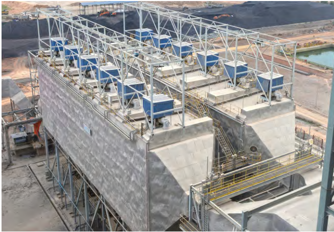
67.5 MW CFBC Power Plant at Bhubaneshwar Power Pvt. Ltd., Bhubaneshwar
