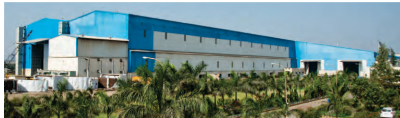
Coastal facility at the port town of Dahej (Gujarat) India with a lifting / handling capacity of 300 MT.
