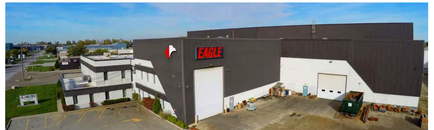
Plant at Windsor (Ontario) Canada for the manufacture of Mechanical Presses.
